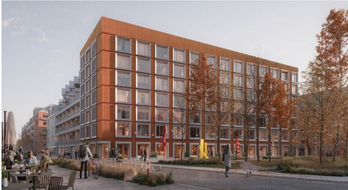
Figure 2. Façade facing the public space. Design by Kaminsky, Mareld, Preservia, Kian Properties, and Moelven.
