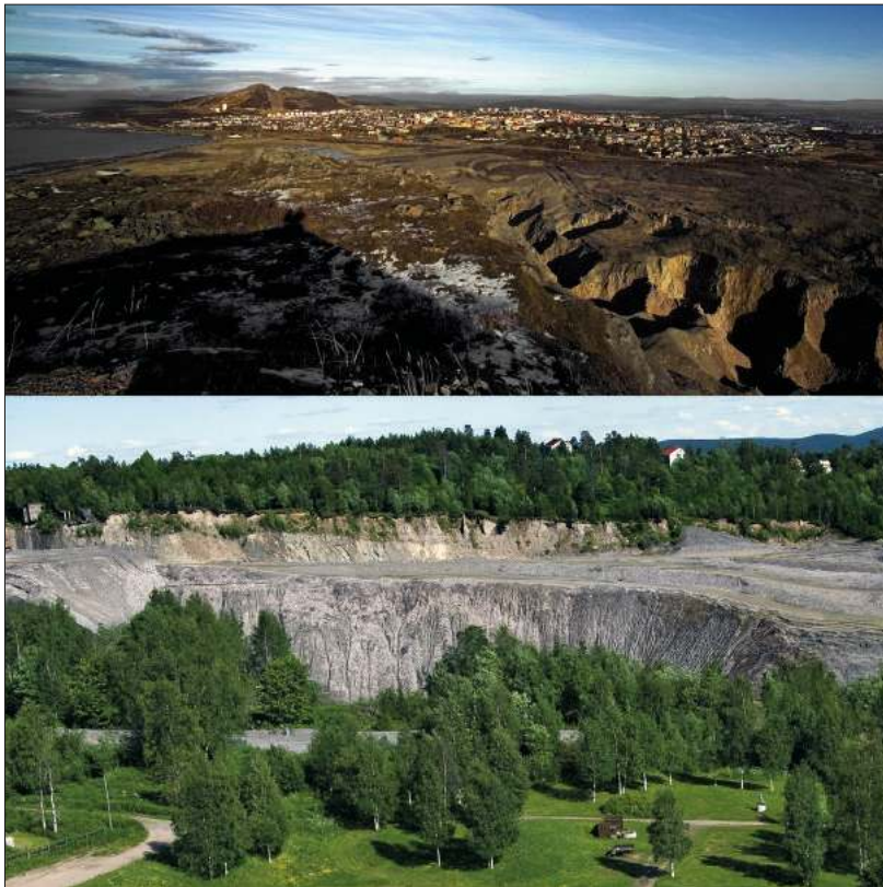
Figure 1. Top image shows Kiruna between the Luossavaara and Kiirunavaara mountains, with subsidence from the mine in the foreground. Bottom image shows the open pit that divides Malmberget. Photo: Daryoush Tahmasebi, Norrbotten's Museum.
