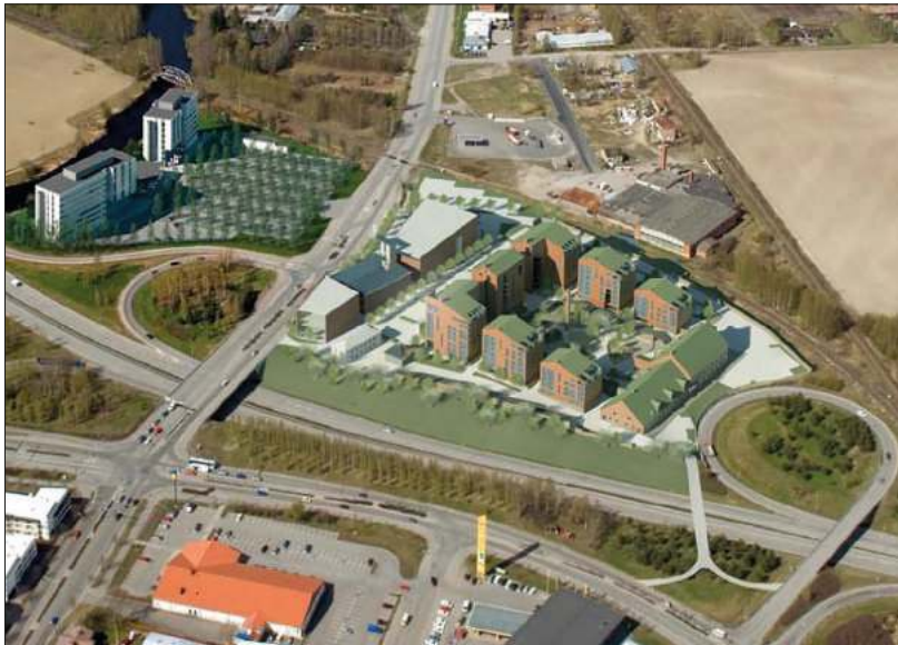
Figure 4. Illustration of Itikanmäki in Seinäjoki. Kalevan Navetta is the low building on the right. Source: City of Seinäjoki.
