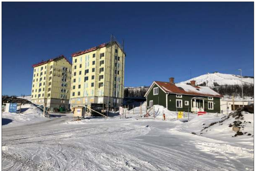
Figure 6. The new company area in Kiruna, with new constructions next to relocated historic buildings. Photo: Jennie Sjöholm.
