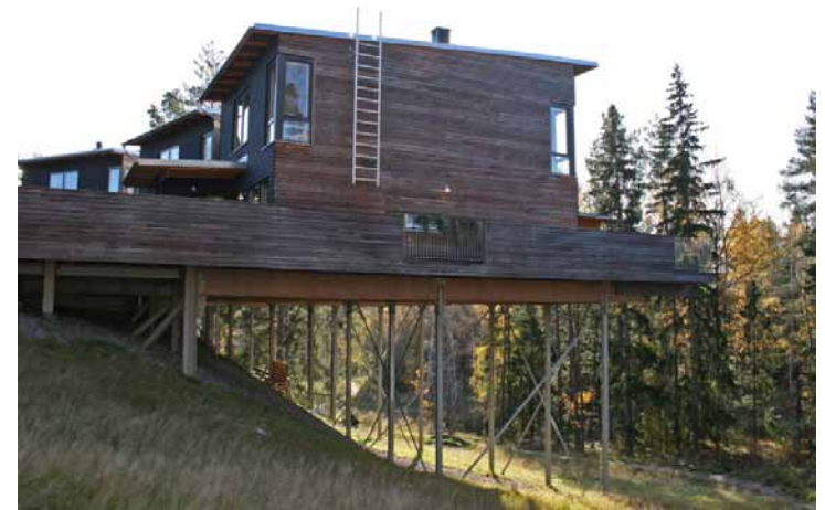
Figure 3. Award-winning wooden-house in Stockholm, Sweden, designed by Brunnerberg & Forshed architect office. Photo by Magnus Rönn, 2011.
